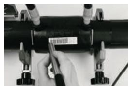
Phase 6 setting up of welding parameters with bar code reader
