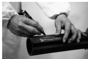
Phase 2 identification of the area to be scrapped
